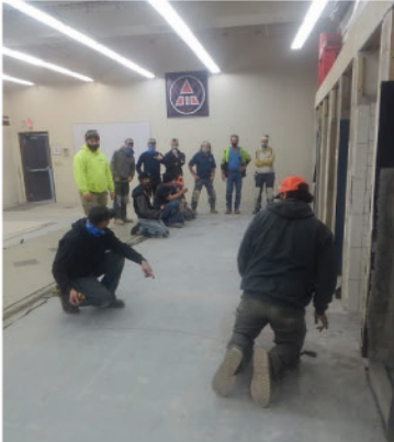
The Greater MN tile apprentices along with their instructors complete floor layout exercises.
