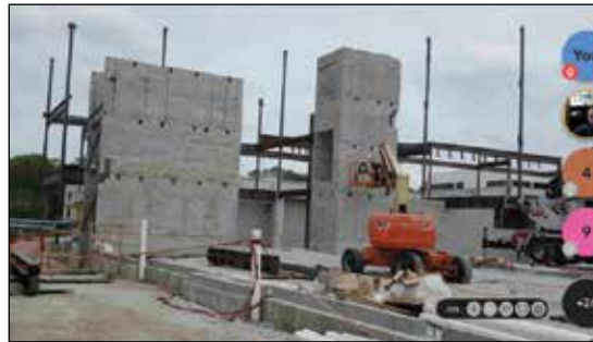
Image of prefabricated stairwells from Sam Rubenzer's presentation to MBJ engineers. For those of you who tuned into the seminar series, thanks for attending. Mark Swanson at IMI, and Rubenzer at FORSE Consulting are available to consult on masonry projects for us, and in many cases at no charge.
