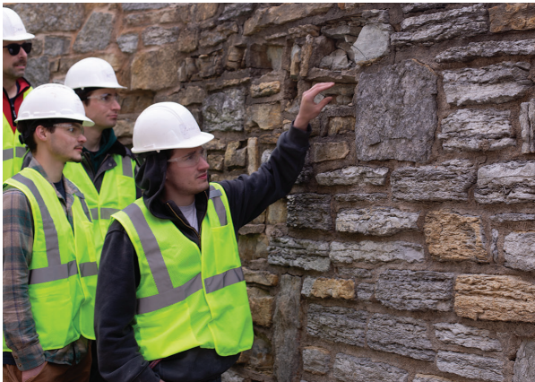
Pre-apprentices take a closer look at historic stonework, discussing the materials and construction techniques visible throughout Fort Snelling.
