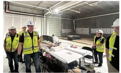
CSI Fargo-Moorhead members review active construction at the Fargo-Moorhead Community Theatre project. Photo: IMI.
