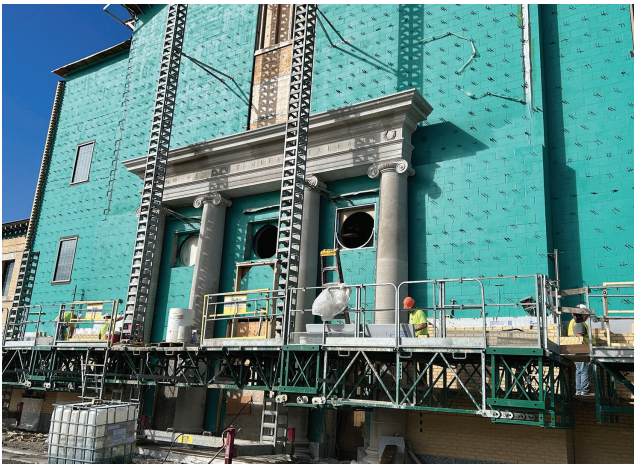
Fargo/Moorhead area members working together on the line installing units on hydro-mobile scaffolding.
